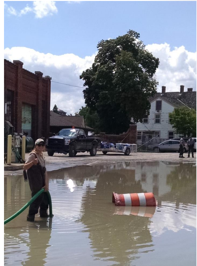
Collapsed Storm line
