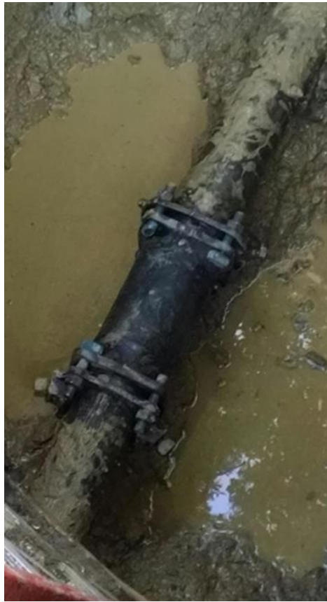
Driving Range Water Mainline Break
