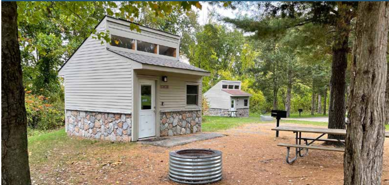
Mini cabins at the campground
