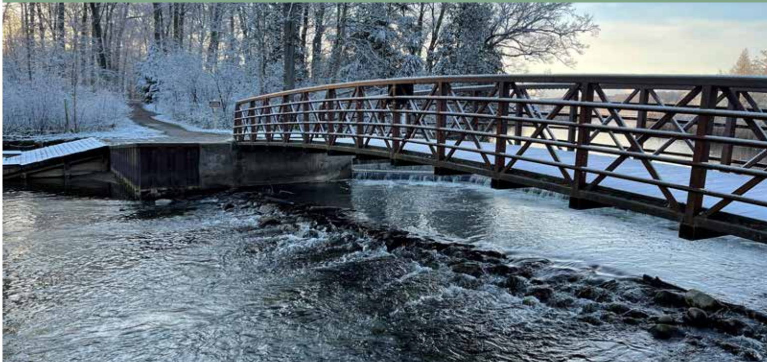
A bridge over the Huron River
